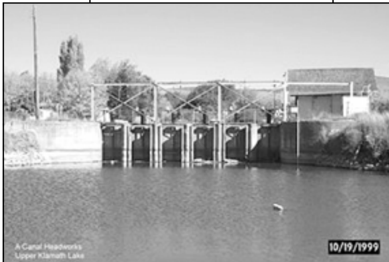
The control gates at the south end of the lake are used to draw off irrigation water.
